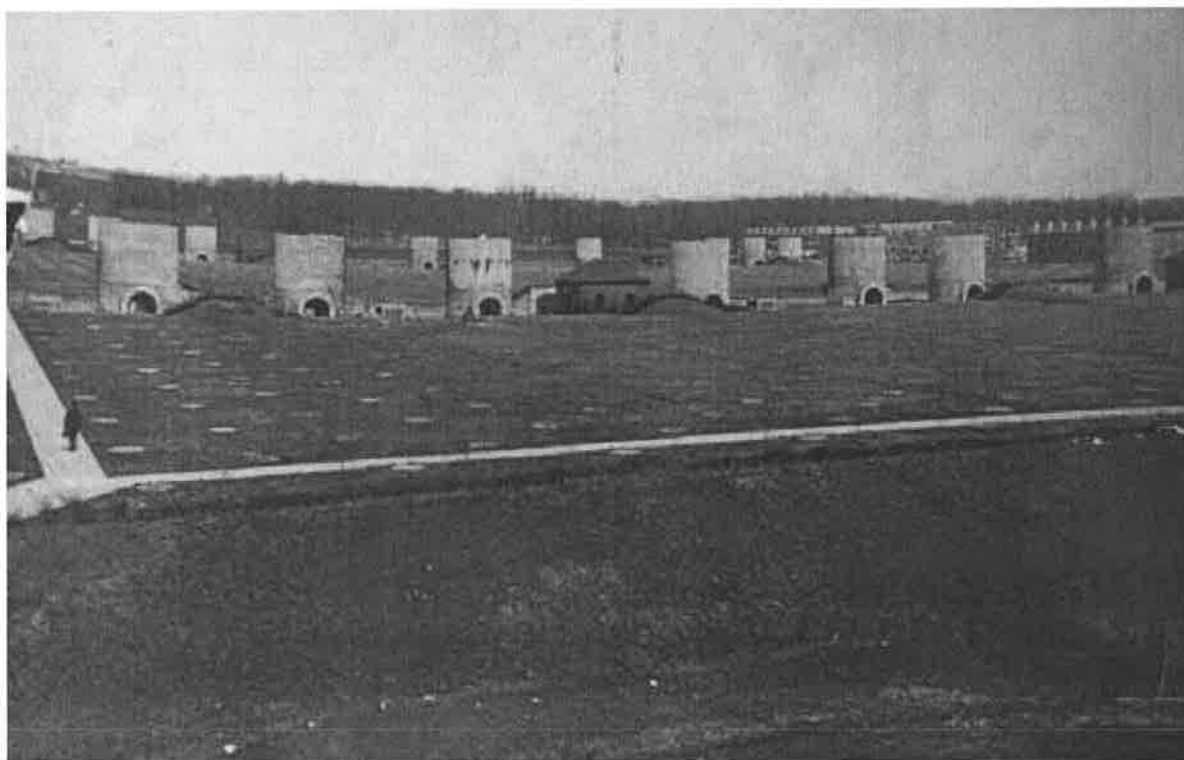
View looking NE over filter beds, ca, 1910
