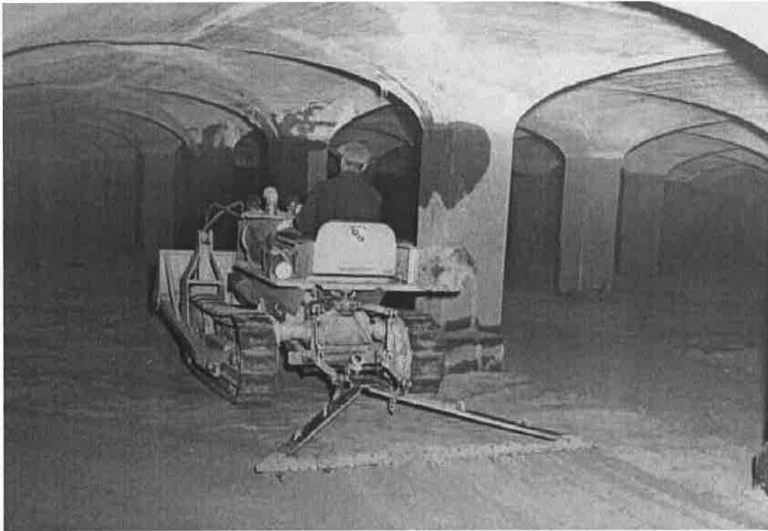
Tractor and filter rake pulverizing the filter sand surface and filter operation (c. 1944) Courtesy of the Archives of the Washington Aqueduct
