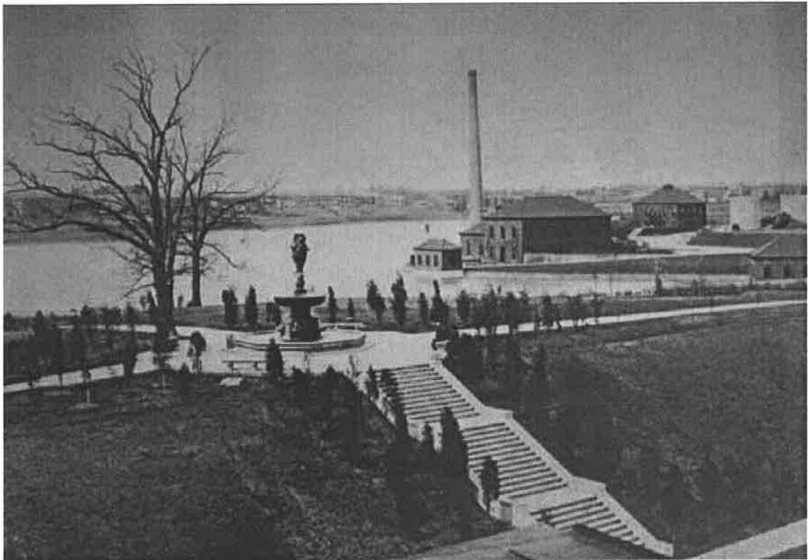
McMillan Memorial, east of First Street near intersection of Channing Street and First Street (c. 1911) Courtesy of the Archives of the Washington Aqueduct
